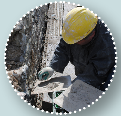
Here, selective pointing is being carried out to facilitate maintenance of access points for bats and birds. Certain gaps can be left without interfering with the structural stability of the building
